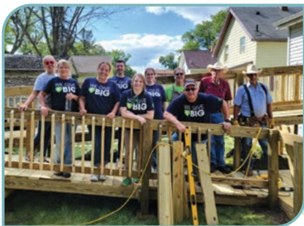
Jackson member center partnering to build a wheelchair ramp.
